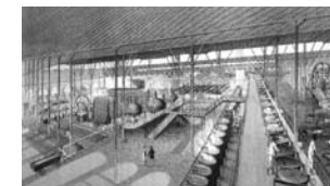
Figs. a and b: Interior and exterior views of the Ingenio Flor de Cuba (Flower of Cuba)
